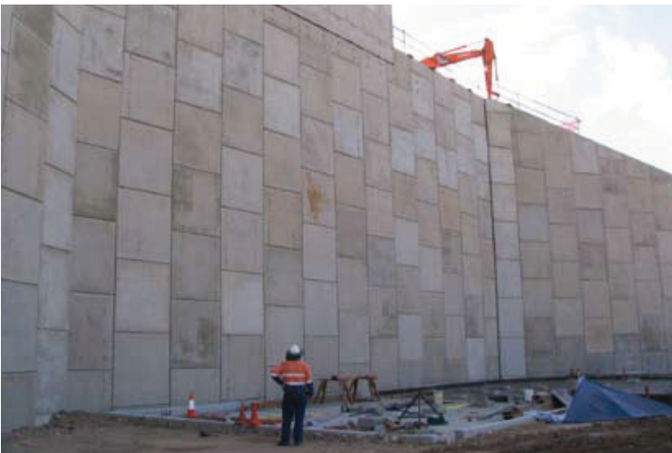
ROM Dump Structure, Bengalla Hine, Australia
